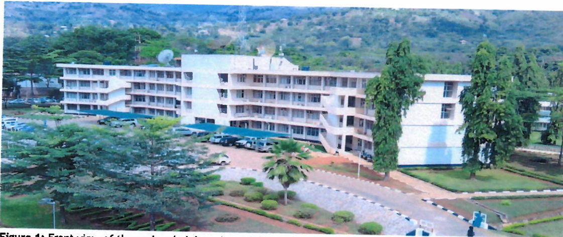
Figure 1: Front view of the main administrative building at Edward Moringe Campus
